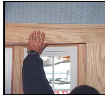
Lightly Sand all Interior Wood Surfaces
