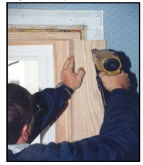
10-i: Fasten 2-1/4" casing to perimeter
