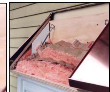
Insulate all Roof Cavities
