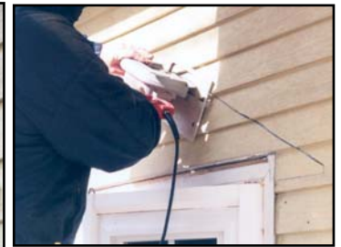
Install J-Channel over siding edge
