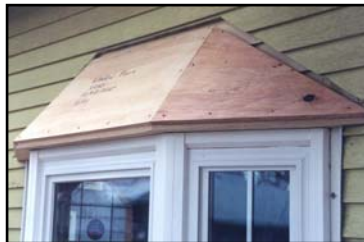
Fasten Roof to Wall and Frame
