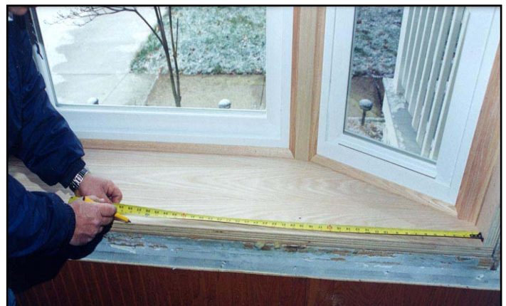
10-e: Measure and Mark Center of Frame and Bottom Face Board
