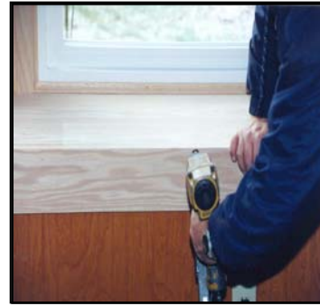
10-h: Top Face Board rests on Sides
