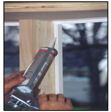
7-b: Insulate between Windows and Frame
