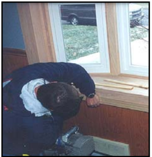
Lightly Sand all Interior Wood Surfaces
