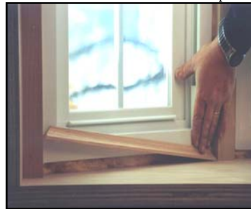
7-c: Install Interior Window Stops
