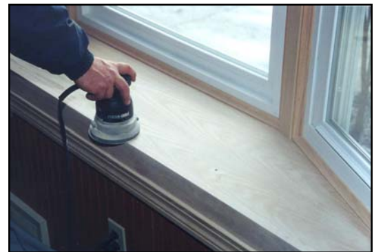
Lightly Sand all Interior Wood Surfaces
