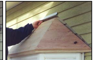
Anchor Upper Eyebolts through Roof
