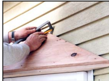
Position Roof Centered on Frame
