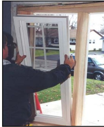
7-c: Install Interior Window Stops
