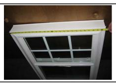
2. Cut Nail Fin to length using a miter saw with a fine tooth blade (Add 3 1/16" to your measurements for outside nailfin cut dimensions).
