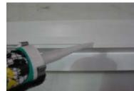
9. Apply sealant and tool the outside face of the joints where all of the nailfins meet and where the nailfin meets the window.
