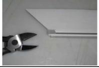
4. Clean out the snap groove so the nailfin will snap in without obstructions.
