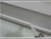
6. Apply a bead of sealant in snap groove of window.
