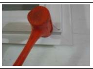
8. Apply a small bead of sealant to the outside face where the fin meets the window to "dress" it up and also as an additional sealed joint.
