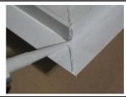
10. Apply a bead of sealant on the backside of the nailfin where the nailfin meets the window and where the nailfins meet along the miter.
