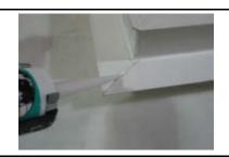
11. Pre-drill 3/32" hole every 6" on each jamb and fill with sealant; then use #8 x 5/8" stainless steel pan head screw and fasten them in the pre-drilled holes. After screws are in place, sealant over the heads of the screws.
