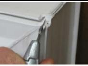
5. Apply a minimum of 1/4" bead of sealant to back side of the snap groove of the window frame.
